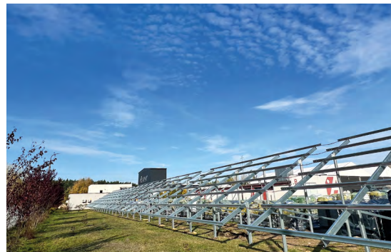
Photovoltaic system in construction in autumn 2022
