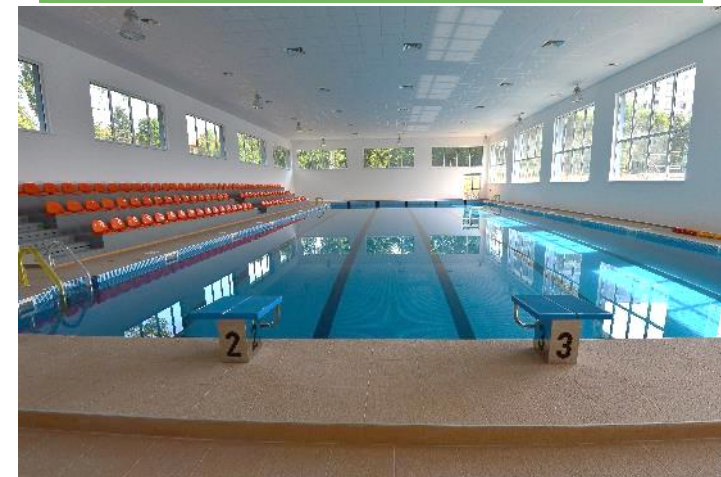
Renovation and EE measures of a swimming pool in the municipality of Pavlikeni
