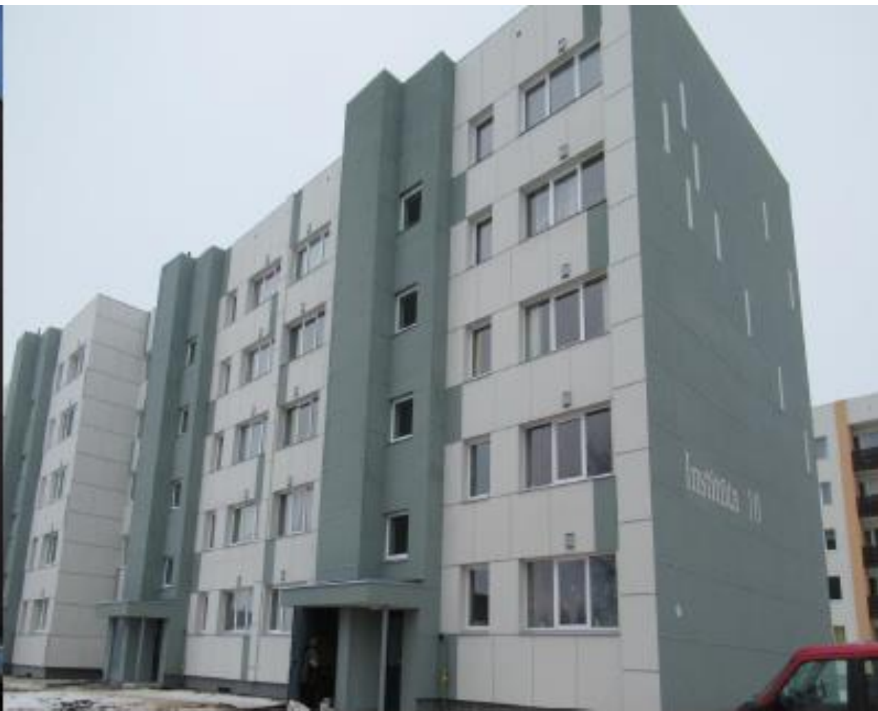
Total cost of project: EUR 778 480 Consumption before: 159 kWh/m 2 Planned consumption after: 52 kWh/m 2
