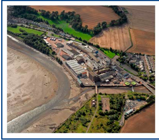
Guardbridge, St Andrews, Fife
